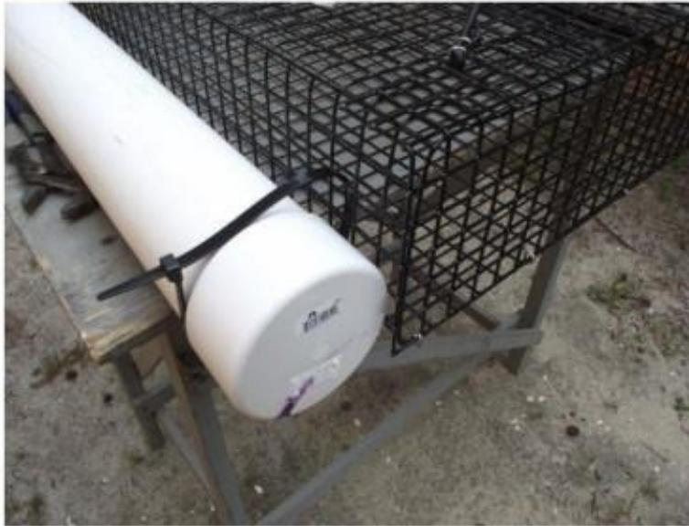
Attach the floats to the sides of the box using 24" or 18" cable ties. The cable ties should be near the ends to keep the PVC floats from sliding back and forth.
