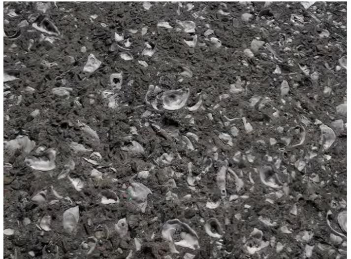
**Example of tabby concrete walls made by the colonists from burning oyster shell which converts the calcium carbonate to quicklime. Shells were also used as aggregate.**
